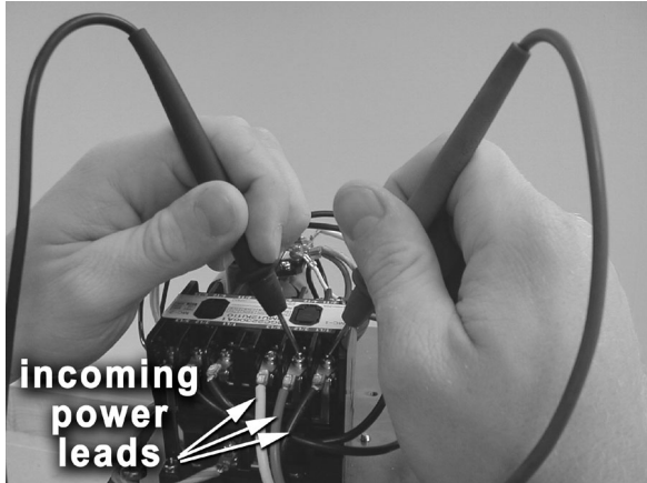
Contactor Voltage Measurement
